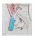
Place the pump and flush tube back in the inside of the water tank
